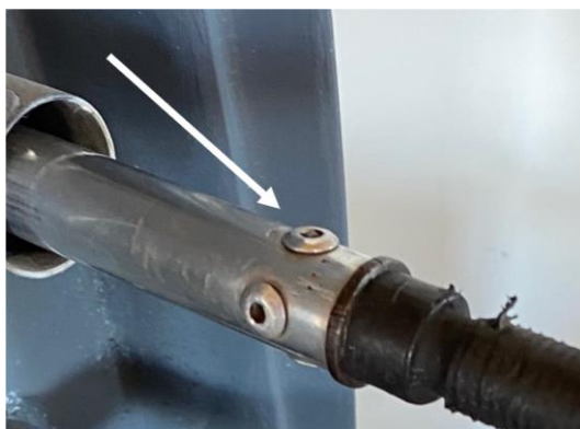
Picture 1: Installation situation old fittings
